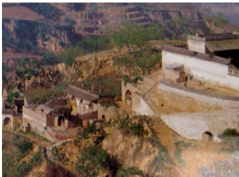
Fig.b The courtyard pattern of cliff Settlement landscape awareness 49
