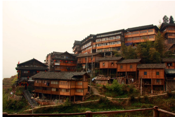
Fig.b Timber structure landscape from the Southwest
