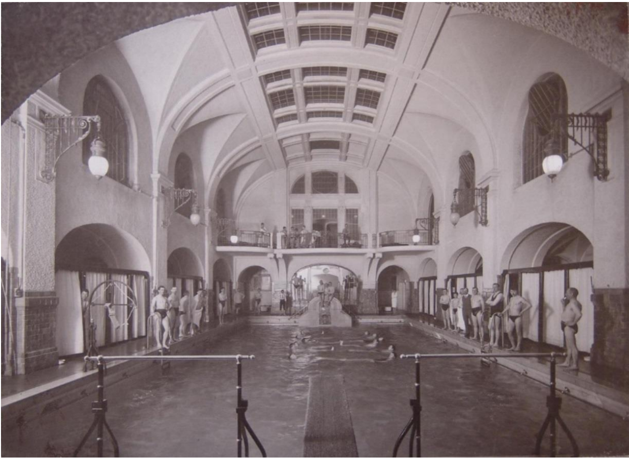
Figure 5: Bertsch (architect) Eduard Züblin (engineer), Municipal bath at Colmar, 1903-1906, (Triboux 2007)
