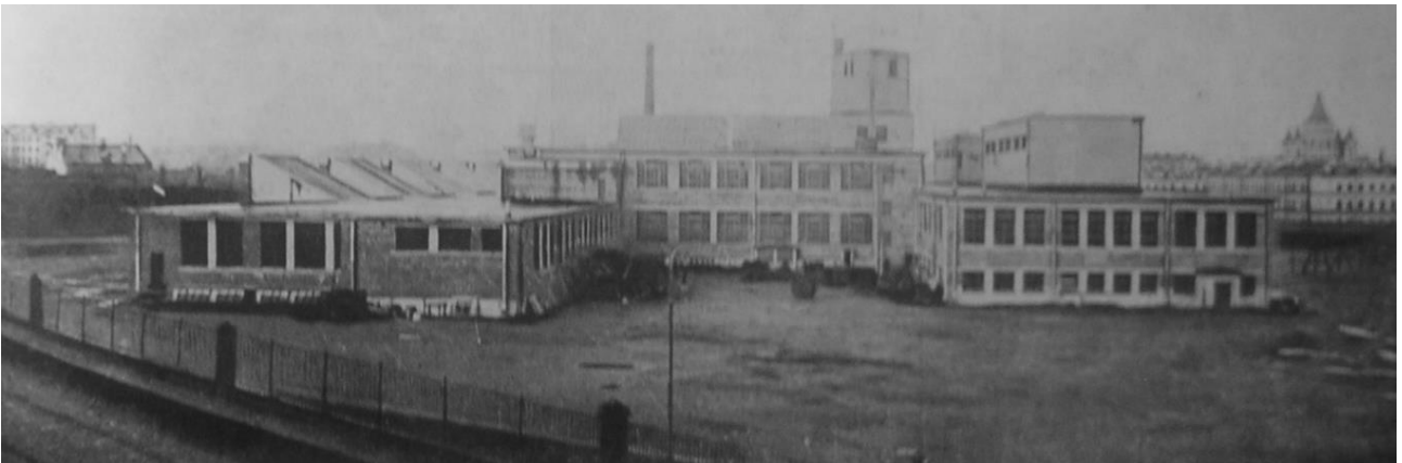
Figure 4: Bread factory "10 years of October" (1926), yard showing H-shape 13
