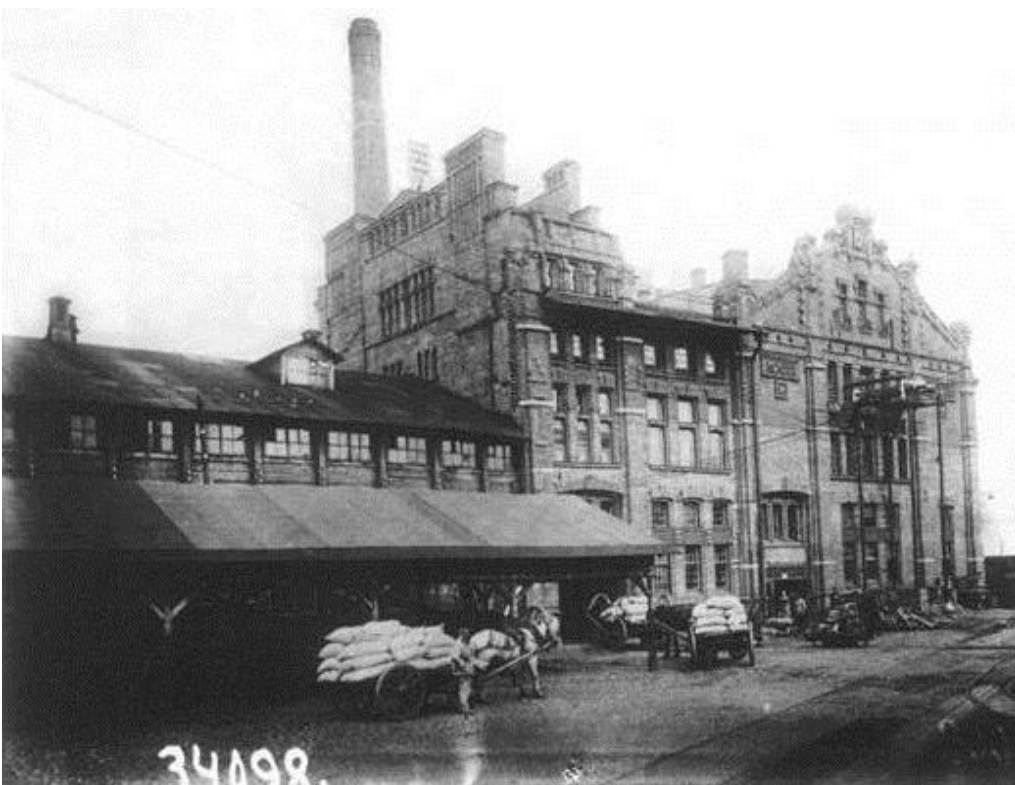
Figure 2: Bread factory Jurgenson, old (1914) wooden part on the left and new brick part on the right 11
