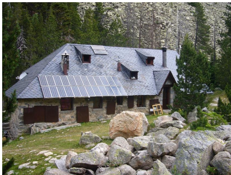
Figure 21 – An isolated mountain hut with stand-alone PV system
