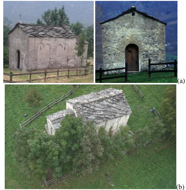
Figure 2.(a) Two detailed view of the S. Maria's Chapel; in (b) it is visible how a part of the object is hidden by trees, which can be a problem for the use of the oblique images to build a part of the complete 3D model
