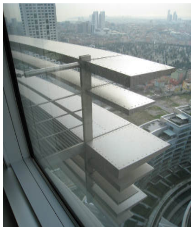
Figure 4.10: Shading devices from inside. Figure 4.11: External shading device drawing detail.
