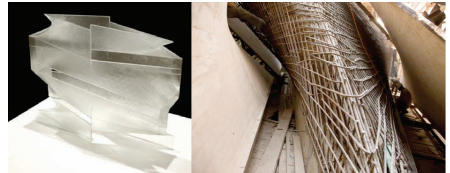
Figure 1. The lightfall: Conceptual model, right. Preparation of wooden formwork and steel reinforcement bars, left. Source: The Tel Aviv Museum of Art.
