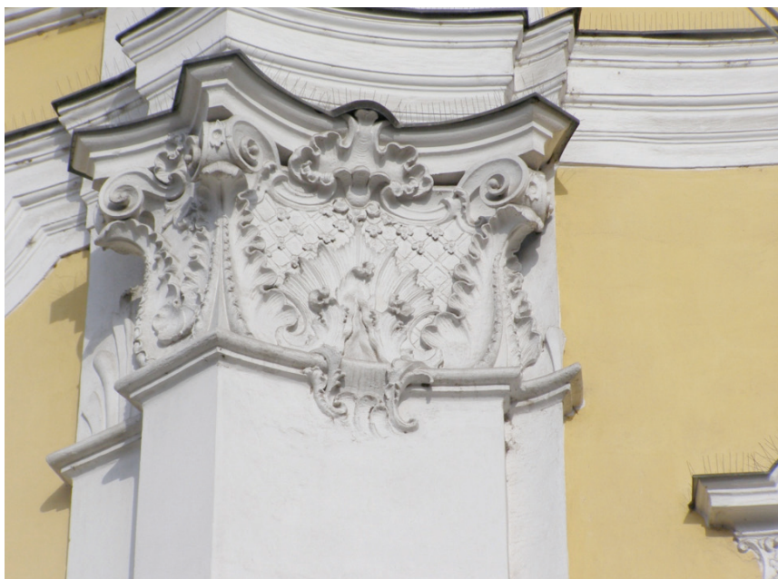
Figure 2. Pilaster capital on the façade of the Barmherzige Brüder monastery church of the Annunciation in Graz, J. G. Stengg, 1735. Source: Photography by Dubravka Botica.
