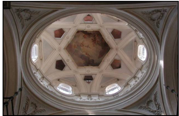
Figure 5 - Removal of the various paint layers;
