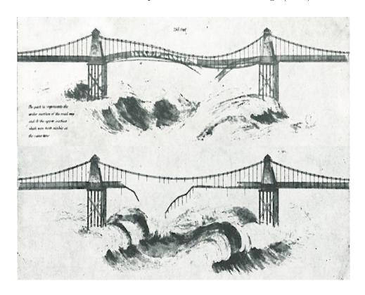
FIGURE 2. Collapse of the Brighton Chain Pier (1836).
