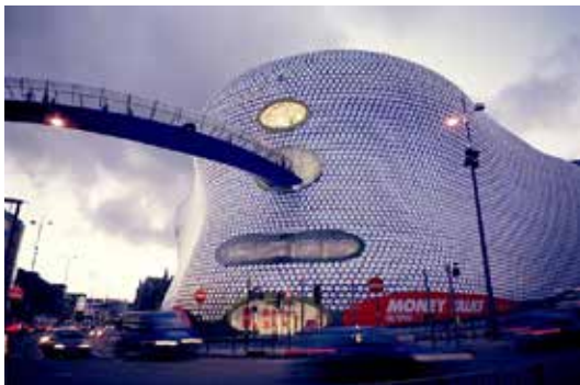
Jan Kaplincky, Selfridges Building, Birmingham 2014.
