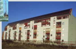
Air solar collector on roof and sun spaces on the south wall
