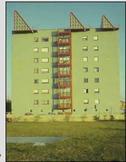
Air solar collector on roof
