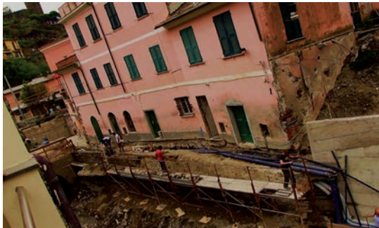
Figure 2.a Flood damages in July 2012.
