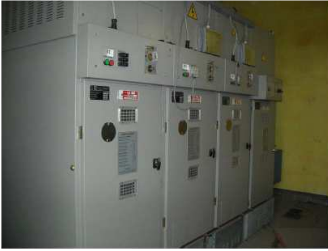
Fig. 6. MV switchgear in the faulted substation.
