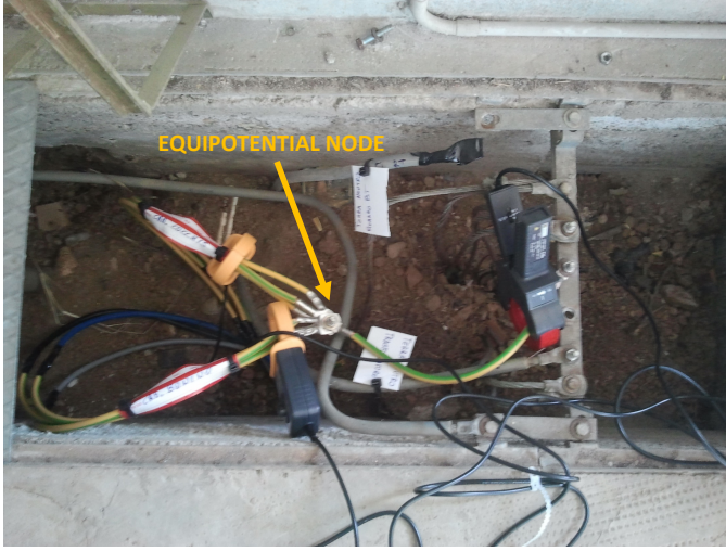
Fig. 5. Equipotential node in the MV/LV substations
