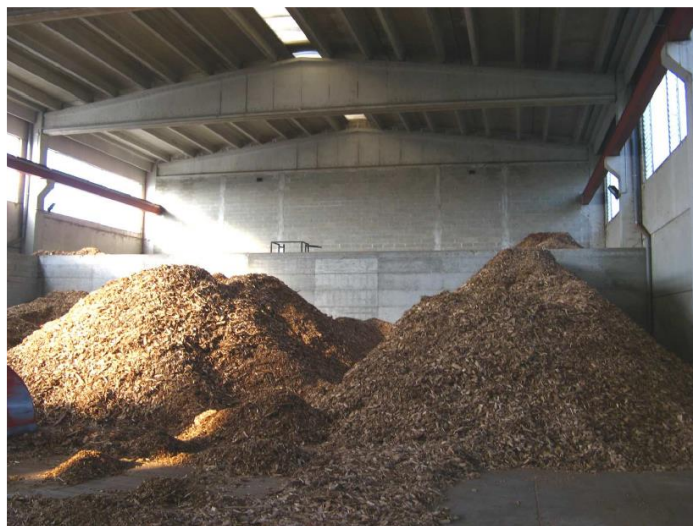
Figure 2.2 Biomass storage in the Leini heating plant
