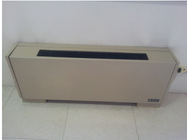
Fig. 3. Example of fan coil unit under examination
