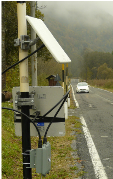
Figure 3.4. Antenna configuration at the RSU: antenna link with CC at the top, and with the OBU at the bottom.
