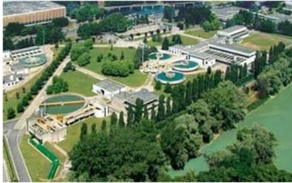
Figure 1-1: Water treatment plant aerial view.
