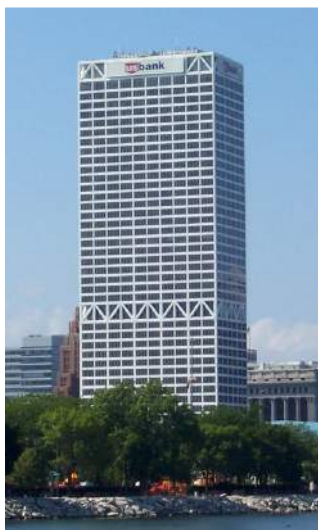
Figure 1.10 – The U.S. Bank Centre in Milwaukee (1973, USA): example of a tall building restrained by two outrigger systems.
