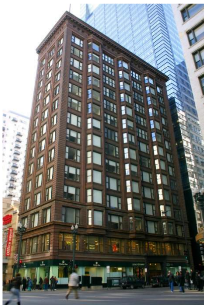
Figure 1.1 – Monadnock Building in Chicago (1981, USA).
