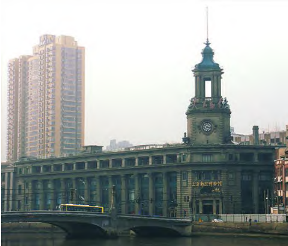
Figure 2-7 New Chinese Post-office and Yangshupu Water Plant, listed as Major Sites Protected for their Historical and Cultural Value at the National Level.(Source: http://zh.wikipedia.org/wiki )
