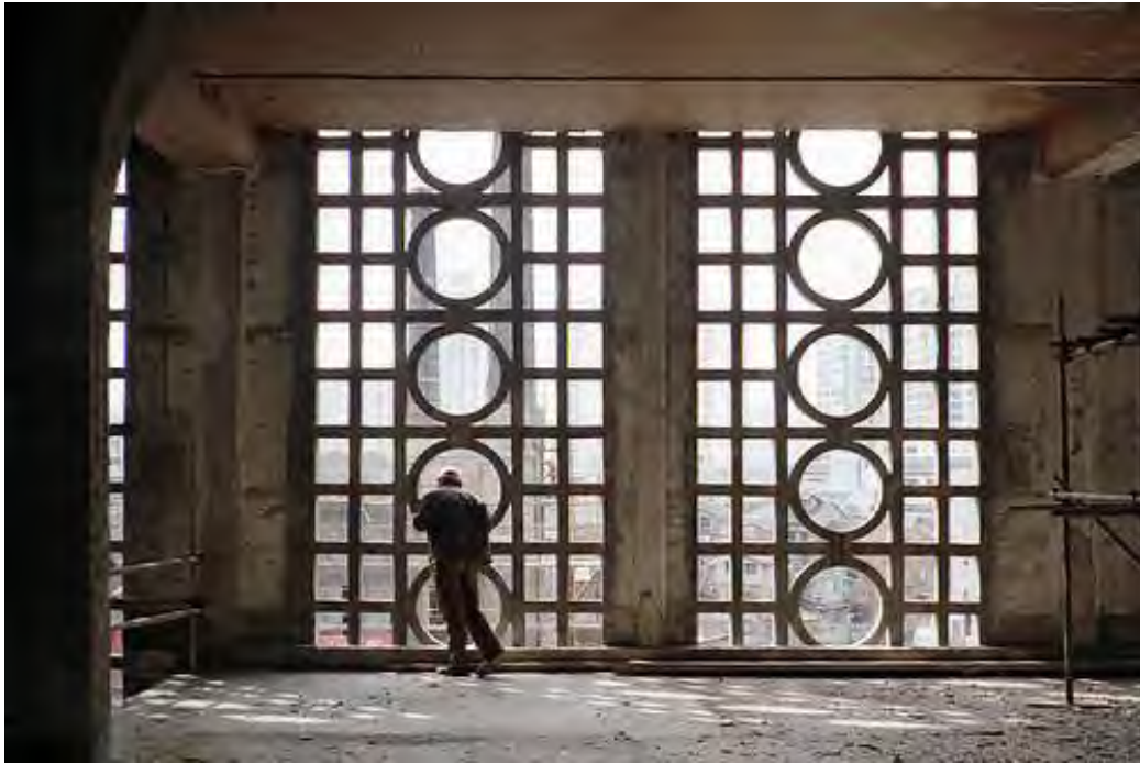
Figure 4-32 The construction site of the restoration project, 2007 (Source: http://forum.xitek.com/forum-viewthread-action-printable-tid-390839.html )
