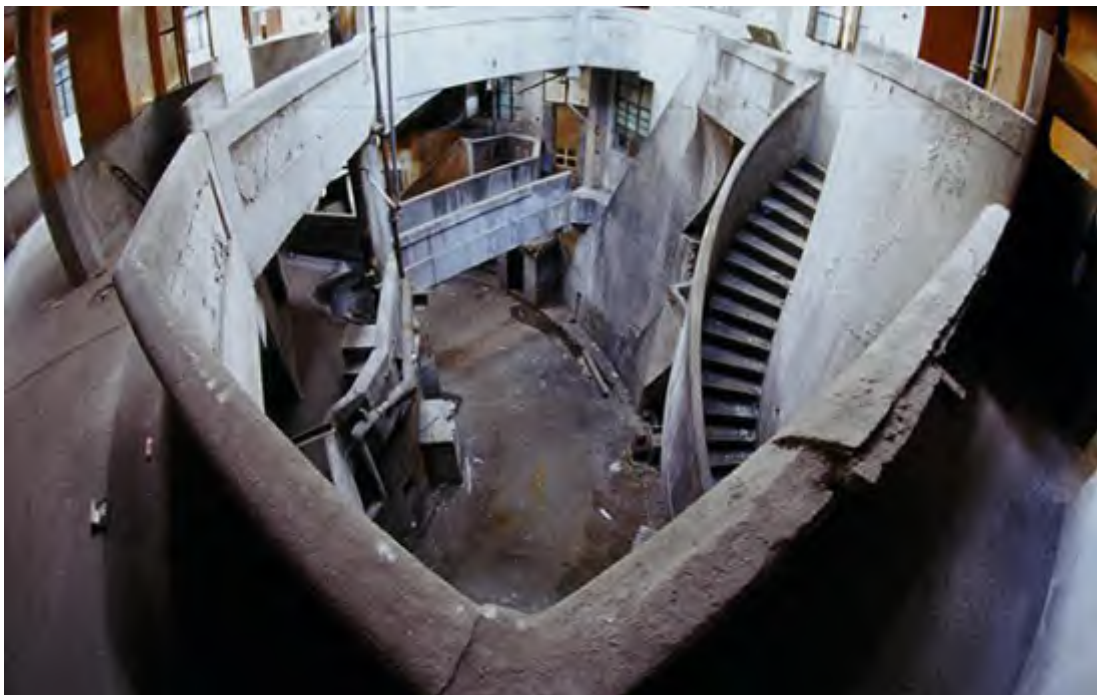
Figure 4-15 The interior of 1# building before the restoration,2006 (Source: http://forum.xitek.com/forum-viewthread-action-printable-tid-390839.html )
