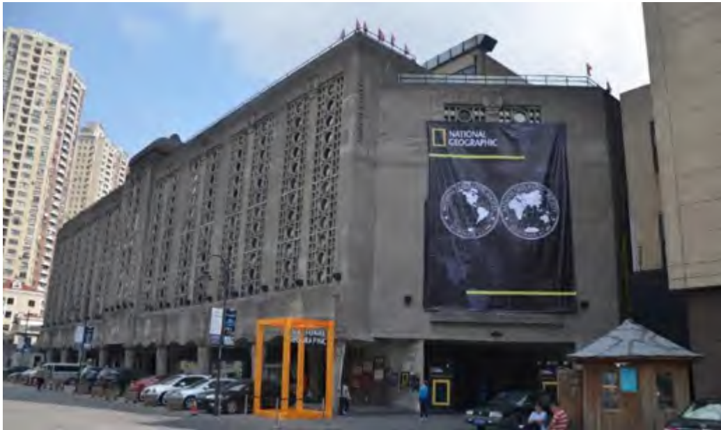
Figure 4-34 The west façade, 1933 Old Millfun after restoration (Photo:by author)
