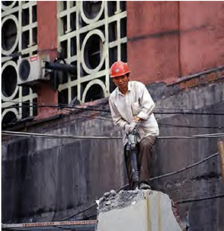
Figure 4-30 The construction site of the restoration project, 2006 (Source: http://forum.xitek.com/forum-viewthread-action-printable-tid-390839.html )
