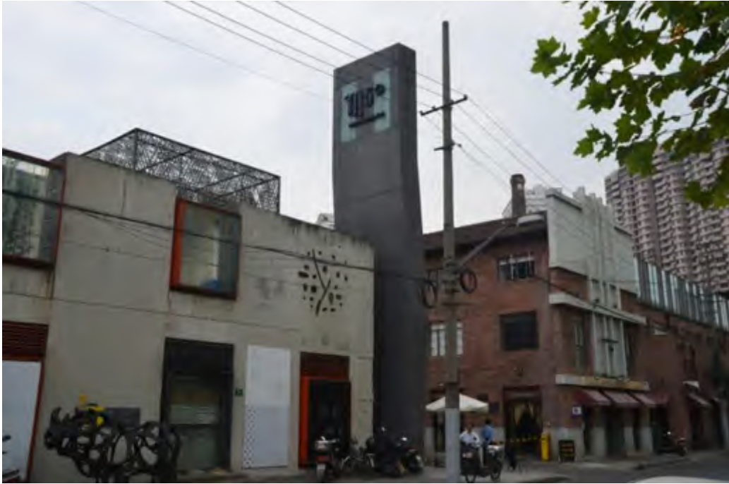
Figure 2-16 M50 on the bank of Suzhou Creek of Shanghai was originally a state-owned textile factory, and rebirthed after an increasing number of artists moved into these old factories. (Photo: by author)
