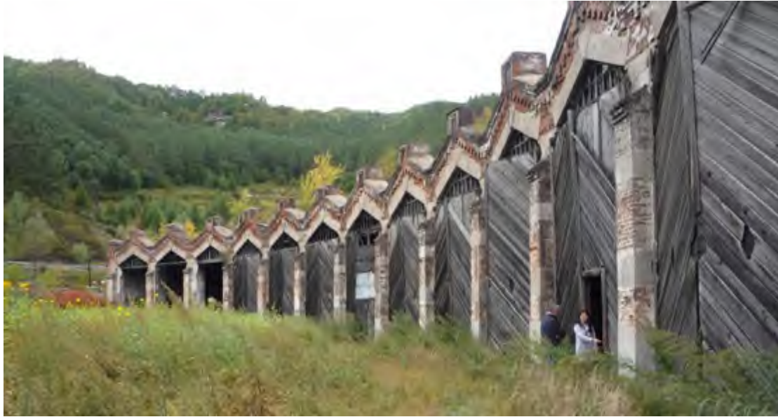
Figure 2-52 View of Locomotive garage of Chinese Eastern Railway in Hengdaohezi .The locomotive garage was built in 1903 and disused in 1990, has a crescent-shaped arrangement with red brick and iron tile. There were 15 parking spaces and a rotary table (already dismantled) in front of the door. (Photo: provided by Marco Trisciuglio)
