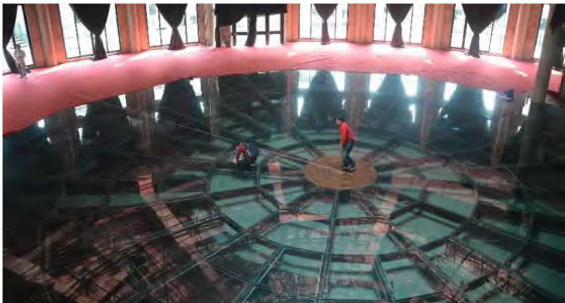
Figure 4-41 The Circular glass floor center hall after restoration, 1# building, 1933 Old Millfun (Photo: by author)
