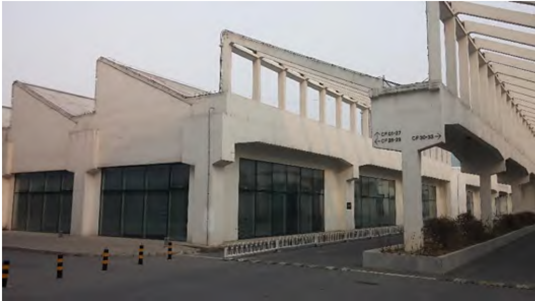
Figure 2-41 Laijin Cultural Creative Industrial Agglomeration Area transformed from Beijing No. 2 Textile Factory (Photo: by author)
