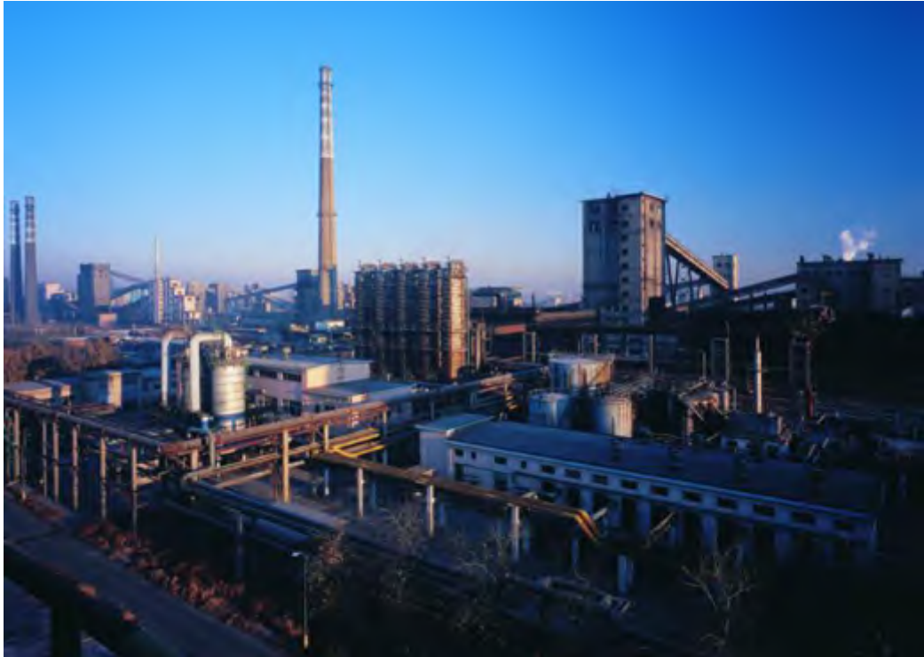
Figure 2-43 Beijing Coking Plant located in the eastern suburb of Beijing (Source: MEN Yu, “The Conflict between Preservation and Revitalization of Beijing Coking Plant”, 2008, 2664–2676.)
