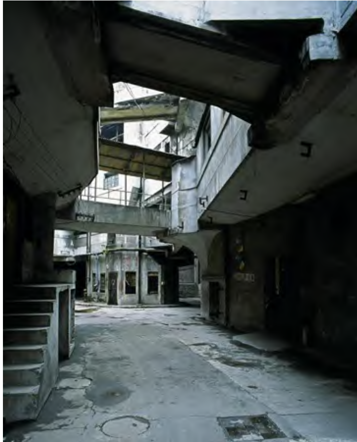
Figure 4-16 The interior of 1# building before the restoration, 2006 (Source: http://forum.xitek.com/forum-viewthread-action-printable-tid-390839.html )
