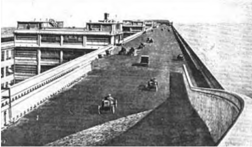
Figure 3-1 The Fiat Lingotto roof with its testing track in action, as published by Le Corbusier in Vers une architecture to illustrate the fusion of engineering, speed and clean structure (Source: Gillian Darley, Factory (Hong Kong: Reaktion Books, 2003), p. 224.)
