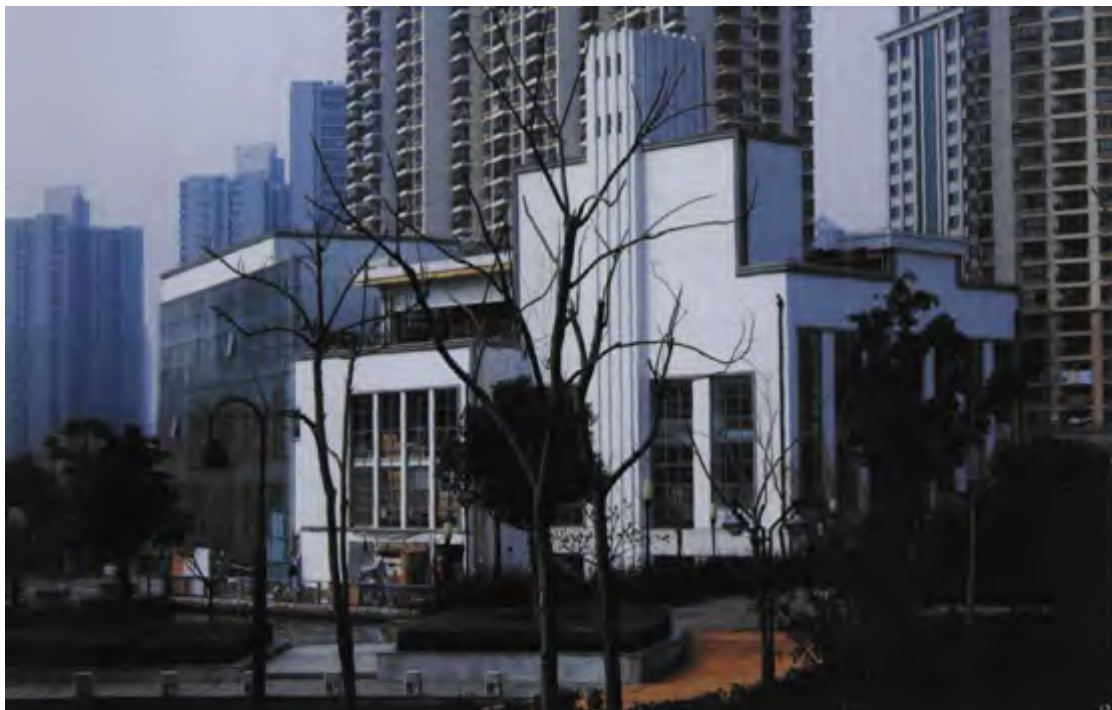
Figure 2-12 General view of the renovated brewing building, now beer bar (Source: Yi-ru, HUANG, and MAO Wei, "Between Demolition and Conservation: Review of the Conservation of the Workshops in Union Brewery Ltd. Shanghai," TIME+ARCHITECTURE, 02 (2006), 88-93)
