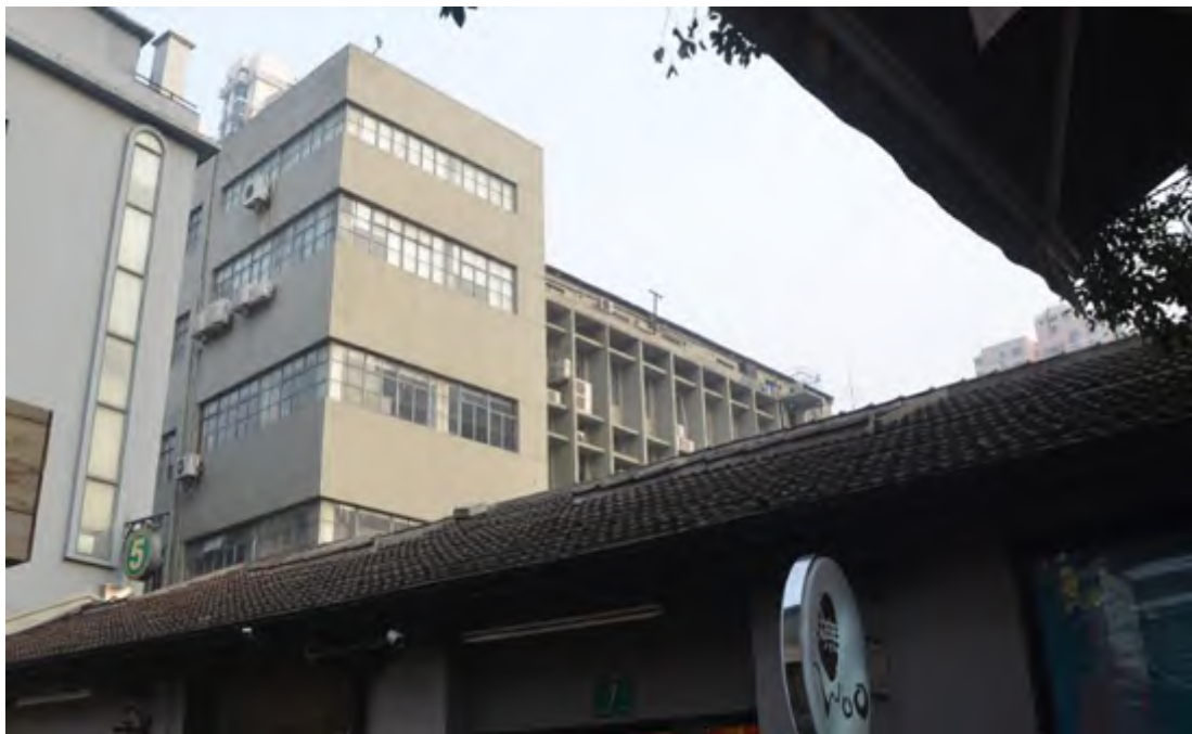
Figure 5-35 The renovated factory in alley 210 (Photo: by author)
