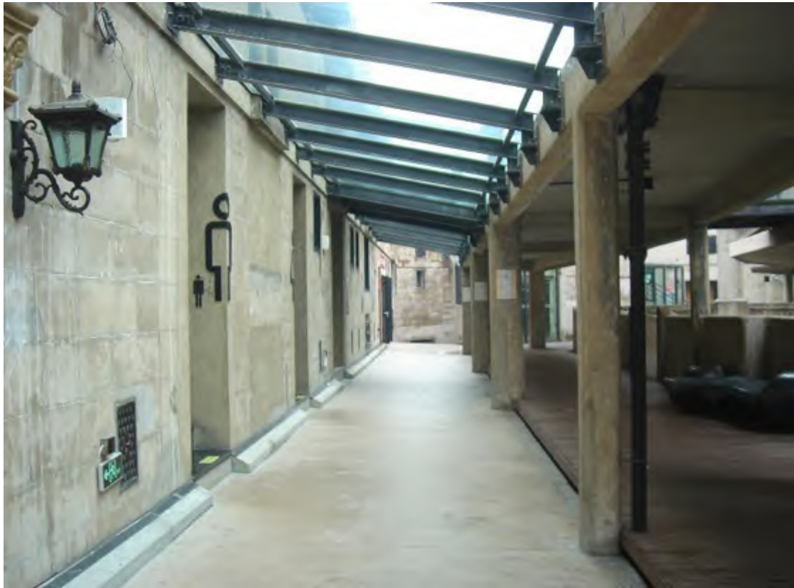
Figure 4-45 The corridors after restoration, 1# building, 1933 Old Millfun (Photo: by author)
