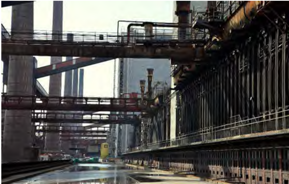
Figure 3-12 Coking plant and the pool(used for ice-skating rink in winter ) in Zollverein, Essen-Katernberg ,Germany. (Photo: by author)
