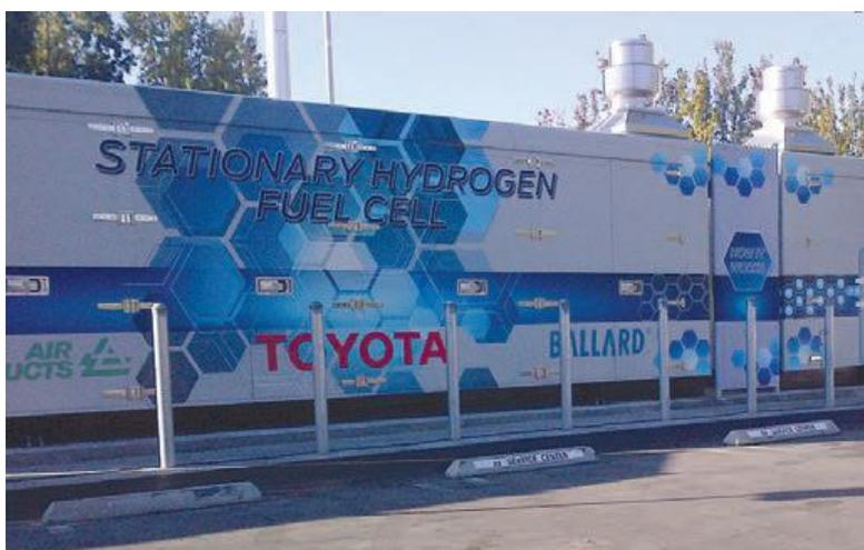
**Figure 1.9.** 1.1 MW PEM fuel cells Ballard system installed at the Toyota Motor Sales in USA [23].
