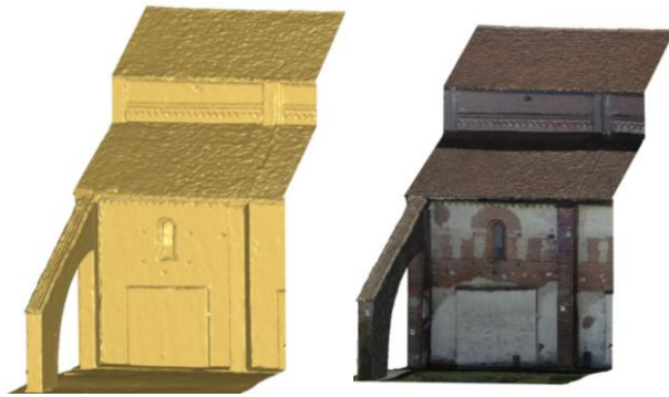
Figure 21. A view of a span of the Church. The mesh has been processed with the “Mesh in two steps” method (distance between points: 0.07 m; deviation error: 0.05 m). The final textured 3Dmodel is on the right.
