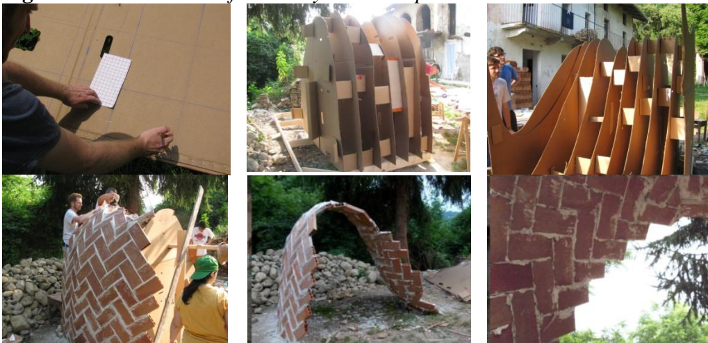
Figure 17. Sequential Steps of Formwork Construction
