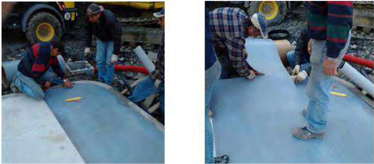
Figure 33 Laying the shielding material
