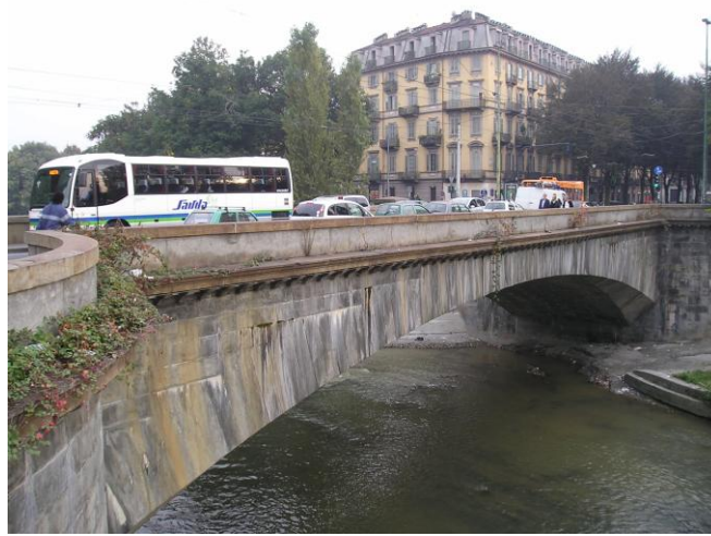
Figure 11. Mosca Bridge under Service Loads.
