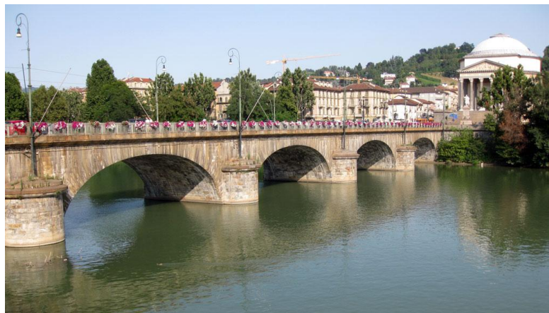
Figure 14. Vittorio Emanuele I Bridge over Po River in Turin.
