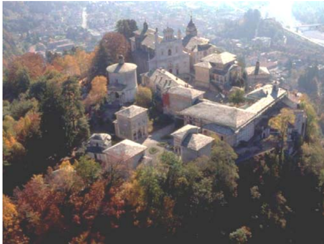
Figure 1: The Sacred Mountain of Varallo, Italy. Overview.
