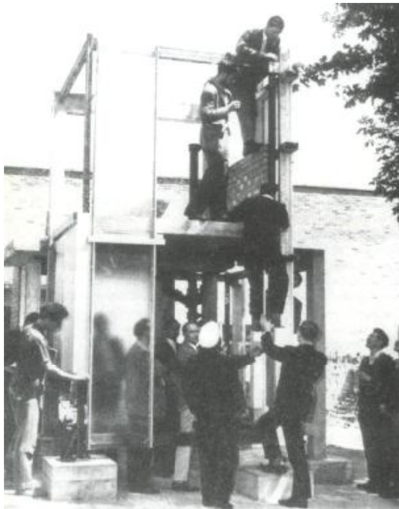
Fig. 22 - Upper school conglomerate - Birmingham School of Architecture 1961
