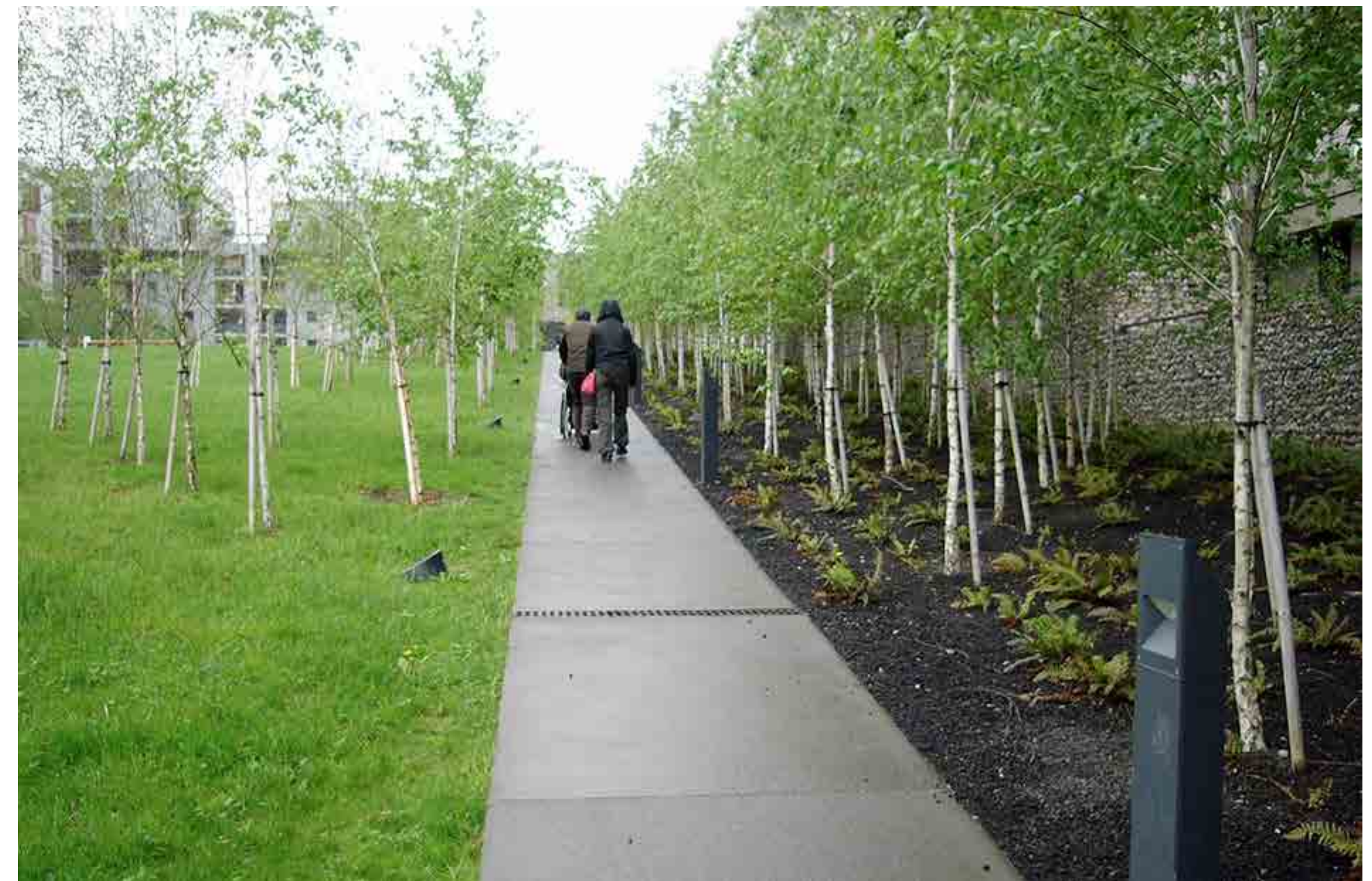
The pedestrian paths with spaces for the soil purification with drainage material and ferns.
