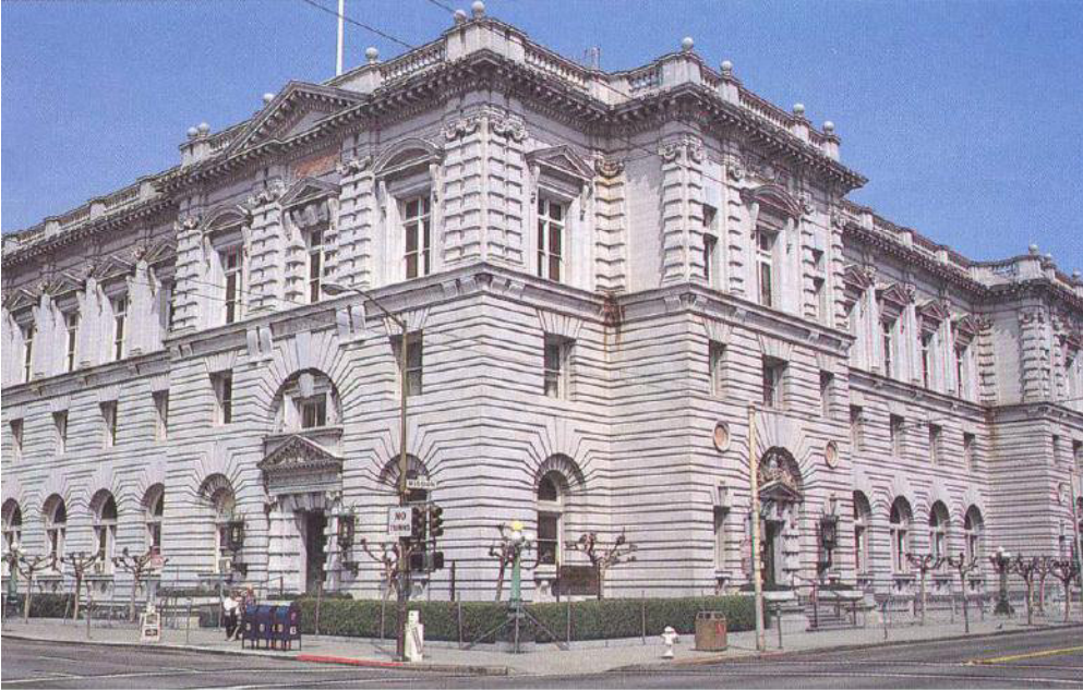
Figure 6: The U.S. Court of Appeals was damaged in the 1989 Loma Prieta earthquake. It is retrofitted with a total of 256 Friction Pendulum Seismic Isolation Bearing, installed between the existing foundation and columns
