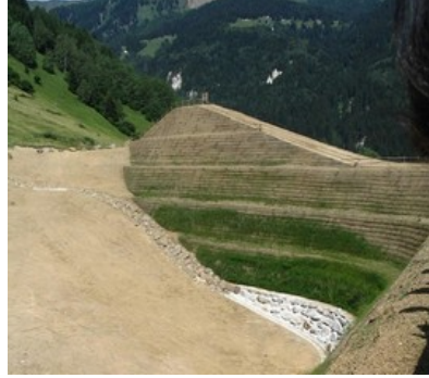
Figure 1.15: Example of a catching dam in Airolo (CH). Photo E. Bovet.
