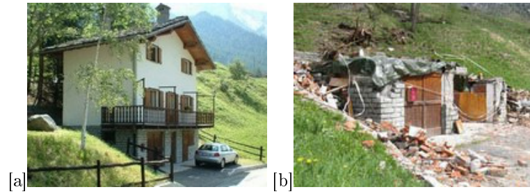
Figure 6.7: Building n.5: [a] before (Photo Rosai) and [b] after (Photo Fusinaz) the avalanche event of 15 th of December 2008.
