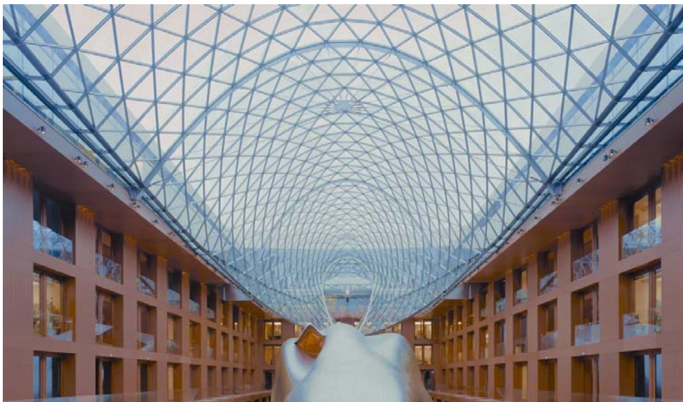
Plate II. Examples of slender structures in a civil contest. Top, Akashi Kaikyo Bridge; bottom, Grid Shell Roof for DZ-Bank.
