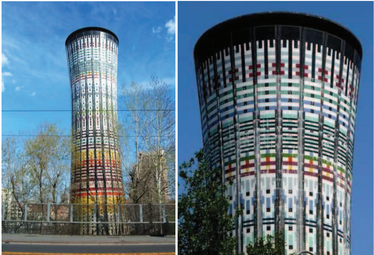
Fig. 6: Water tower near the Farini Bridge at Porta Garibaldi Rail Station, Milan in the new restyling. Restored for the FIFA Football World Cup "Italia'90", the coating is composed by ceramic tiles. (Image from www.panoramio.com ).
