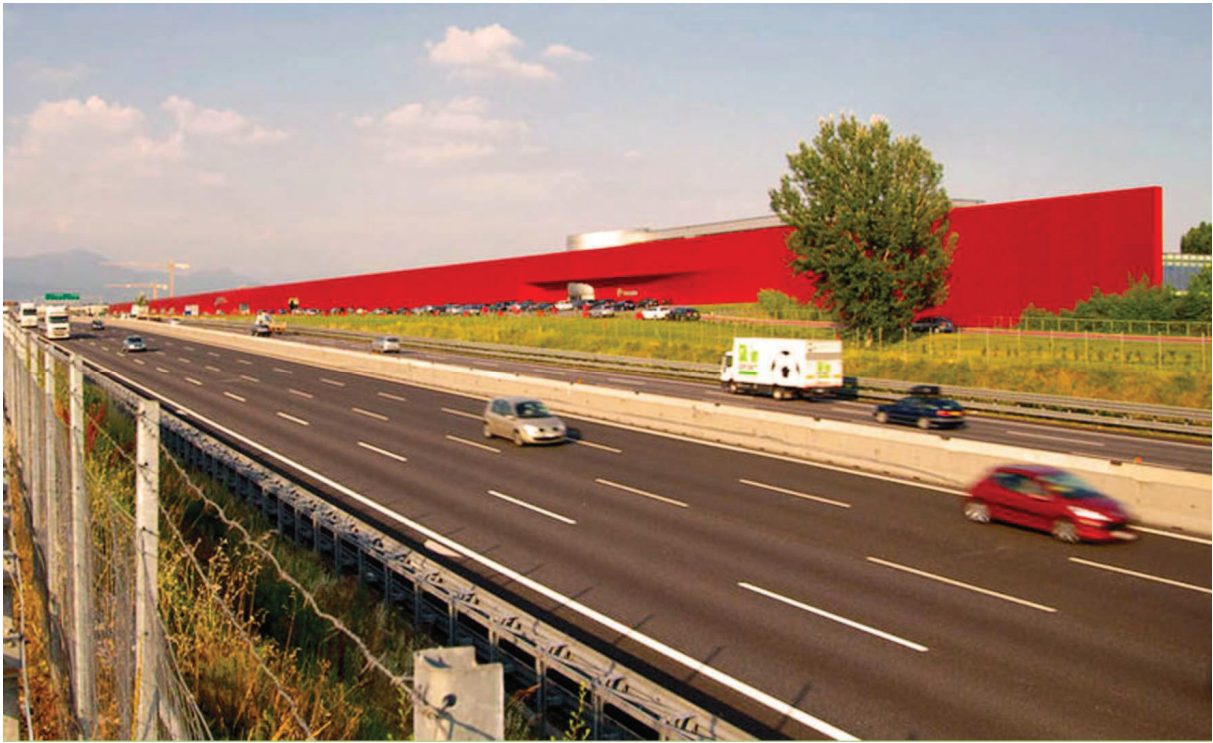
Fig. 3: The Kilometro Rosso seen from the A4 highway. Despite the cars slide quickly down the stretch of road, the perception of the building is guaranteed by its color. The Kilometro Rosso is the first Italian work of the French architect Jean Nouvel; the barrier, which acts as a filter between the highway and the park, is covered extruded aluminum and is just one kilometer long and has an height of 10 meters (da http://www.kilometrorosso.com ).
