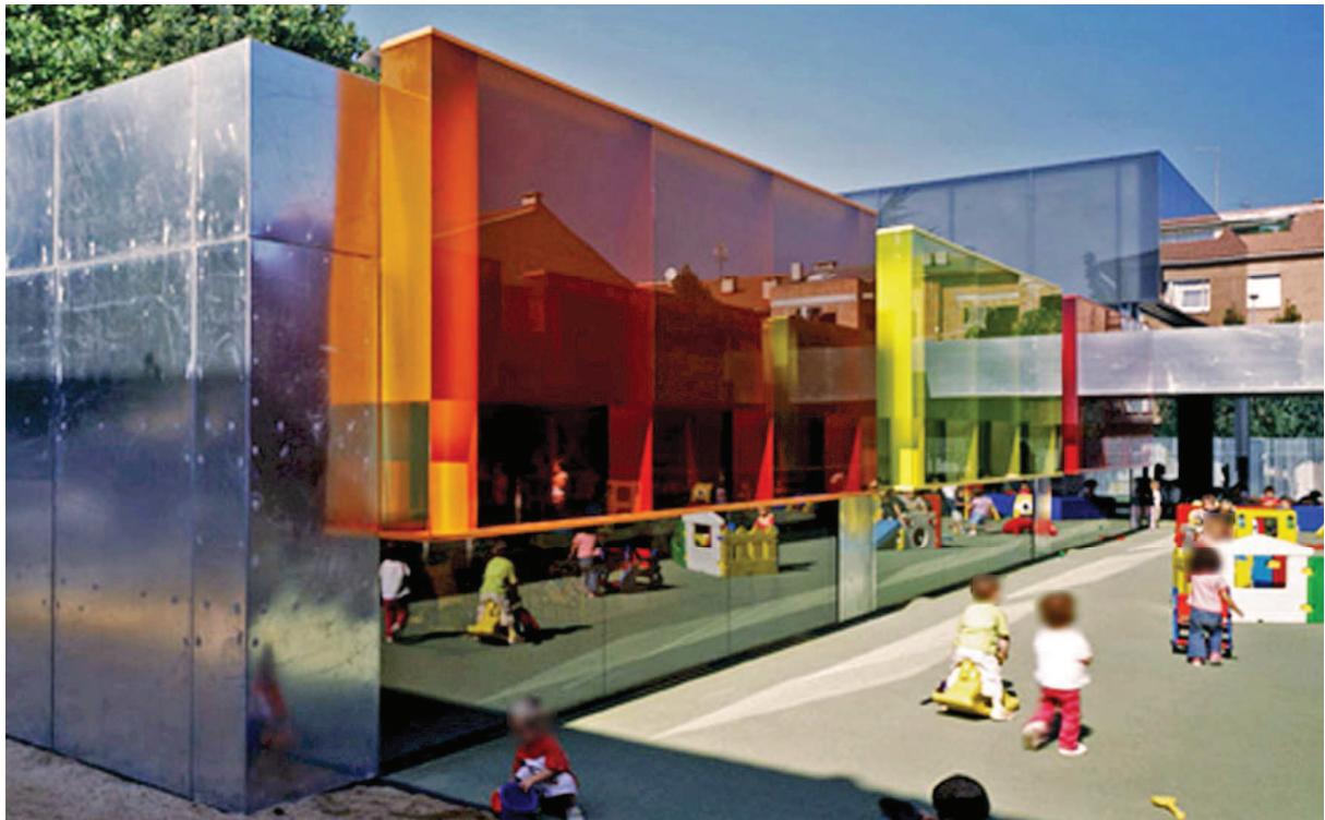
Fig. 1: The interior elevation of asylum that overlooks on the courtyard, used as a recreation area for children. From a technical point of view appears to be _ fundamental the choice of safety glass, due to the proximity of the children to the panels . Colored PVB interlayers provide an ideal level of safety for cases, due to the excellent adhesion to glass and high elasticity, which allows for an effective energy-absorbing shock. (In AA.VV. Asilo Els Colors , The Plan, n. 15, luglio/agosto 2006, p. 63).
