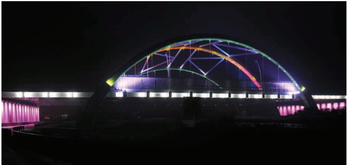
Fig. 5: Centropadane Bridge near Brescia. The lighting design of the bridge is made entirely with LED products, because this technology enables highly dynamic nature and the ability to configure different scenes in an elastic way (da http://www.lighting.philips.it/projects/italian_projects/ponte_centropadane.wpd ).
