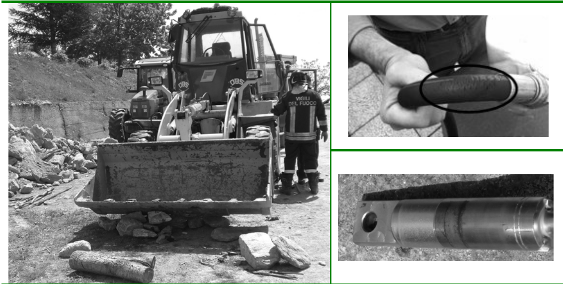
Figures 4.5, 4.6, and 4.7: The machine involved into the event, the poor condition of the broken hose and the worn distributor parts
