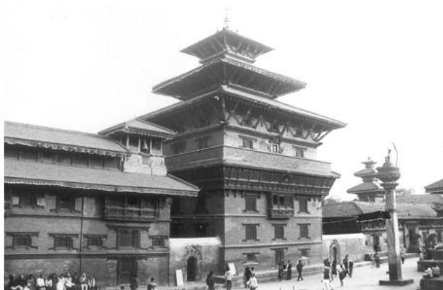
Figure 2.19 - Degu Taleju Temple. Top: This large building with huge wall thickness collapsed completely. Bottom: Contemporary view after reconstruction.
