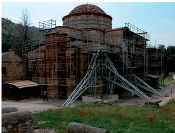
Figure 2.12 - Emergency intervention after the 1999 earthquake at the monastery of Daphni.
