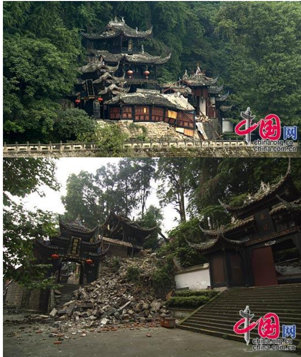
Figure 2.17 - Damage occurred to the Er Wang temple after the Sicuan earthquake in 2008 (Magnitude 7.9).
