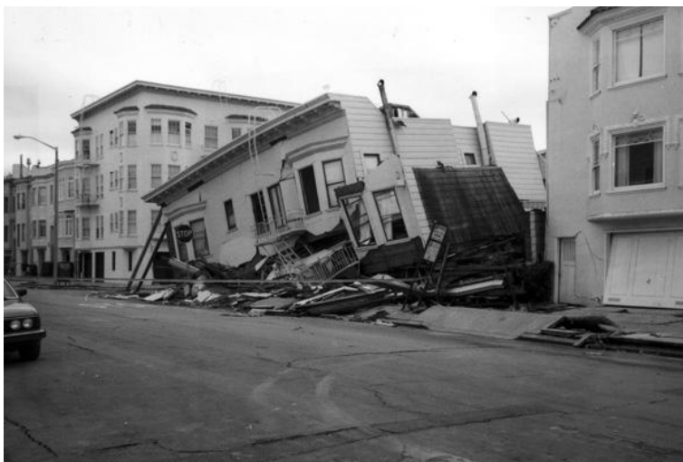
Figure 2.5 - Structures damaged in the Marina District of San Francisco following the Loma Prieta earthquake. The first story of this three-story building was damaged because of liquefaction; the second story collapsed. What is seen is the third story (Credit: Plafker, G, Figure 24B, U.S. Geological Survey Circular 1045).
