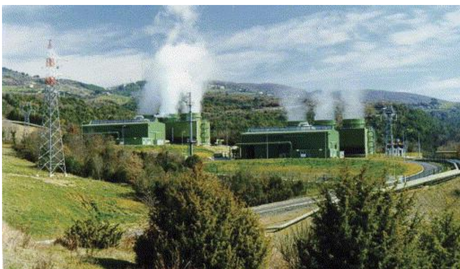
Figure 1.3 Larderello geothermal plant
