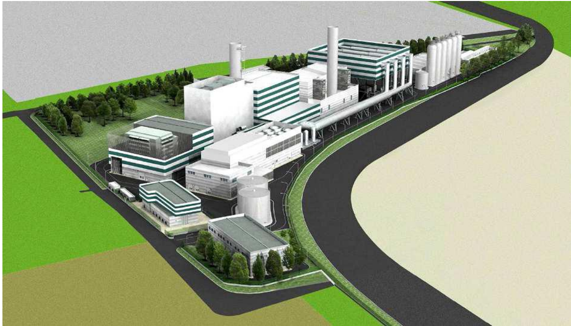
Figure 1.5 The CHP power plant of Torino Nord
