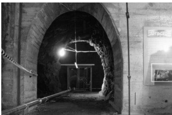
Figure 5. View of one of the vacuum pipes hosting the laser beam of a ring-laser in the Cashmere cavern near Christchurch, NZ.
