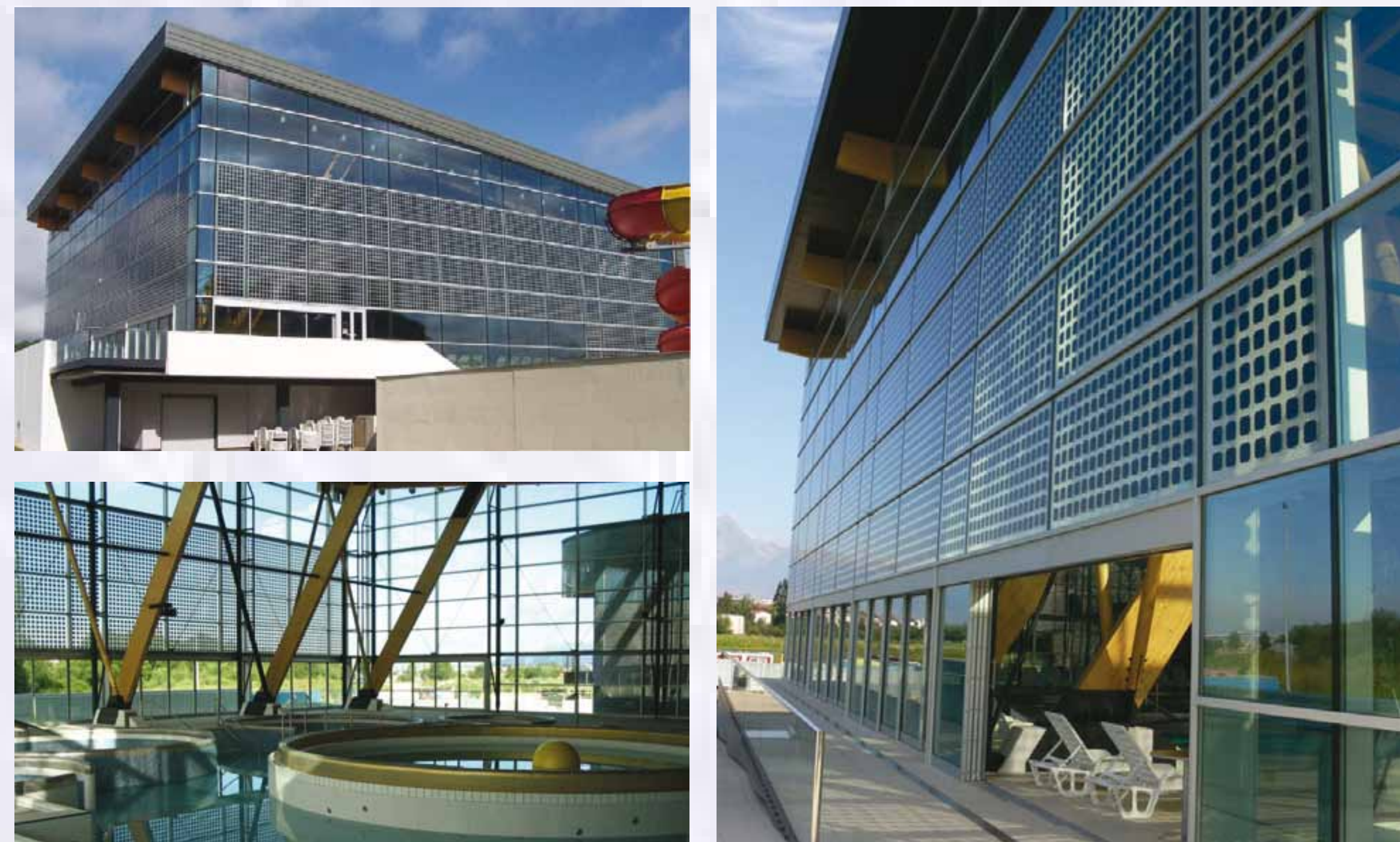
AquaCity Poprad - Aquapark, Slovakia , authors: P.Kučera, F.Rubáš, ARCHSTUDIO (CZ), Relaxation Pool Sapphire Blue, 2007 (fi. Ingsteel, Schuco International, Solarklima)
