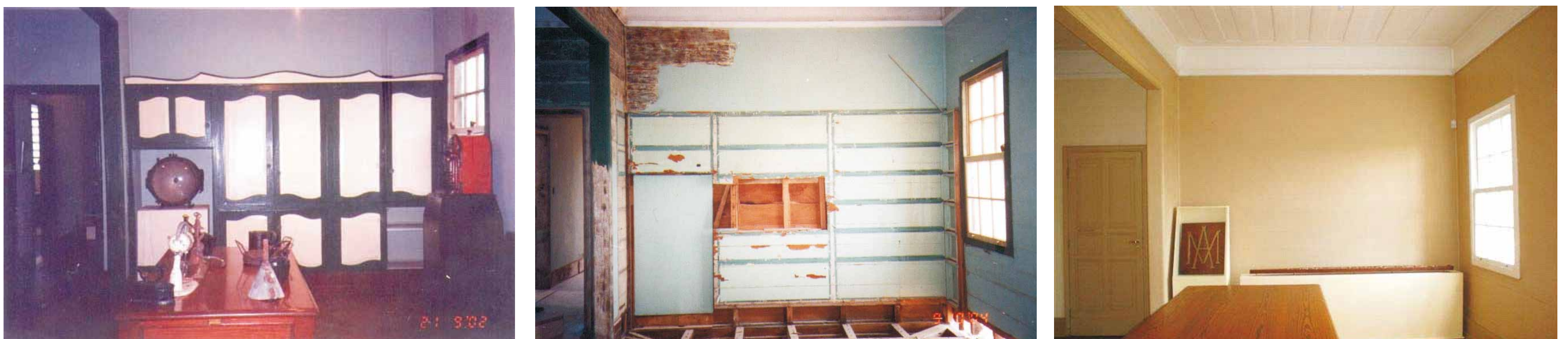
Ambient: pantry. Before, (2002). During, (2004) and after (2012)
