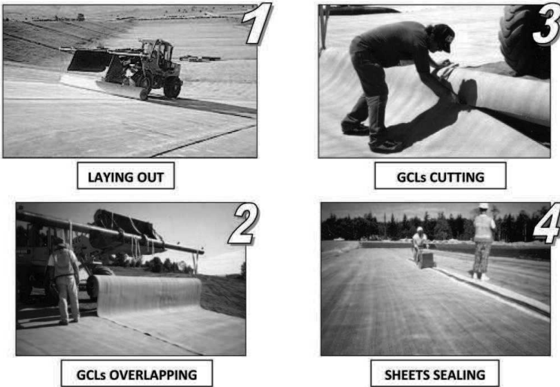
Figure 6.1 – Main installation phases of a GCL in a landfill cover or bottom liner.
