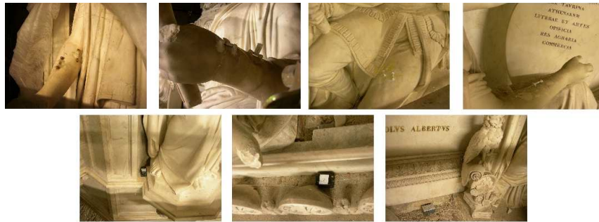
Figure 4.10. Installed measurement nodes and fixed POF displacement sensors on the marble statues inside the chapel during the restoration works.
