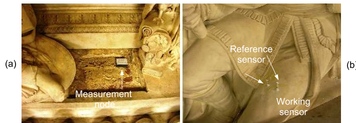
Figure 4.11. Example of one installed measurement node (a), controlling two POF sensors fixed on a female marble statue maintained inside the chapel during the restoration works.
