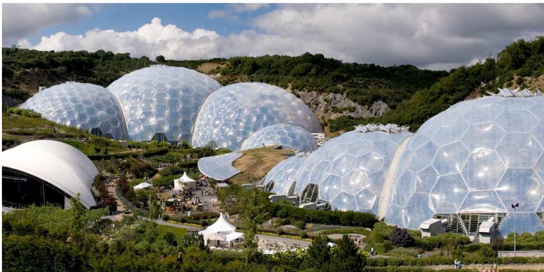
Fig. 154 – NICHOLAS GRIMSHAW, Eden Project , Saint Austell (Cornovaglia) 2011.
