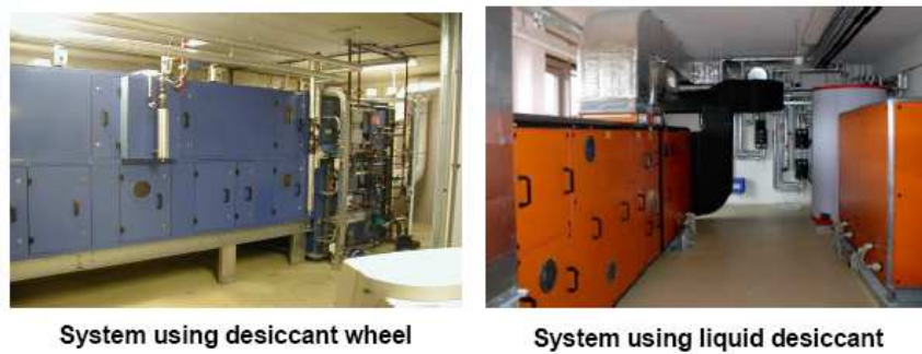
Figure 60 Open cycles-desiccant air handling units
