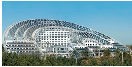
Figure 9 Sun-Moon Mansion in China Solar Valley in Dezhou, Shandong Province, China
