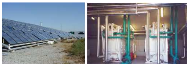
Figure 10A cosmetics factory using solar cooling system near Athens
