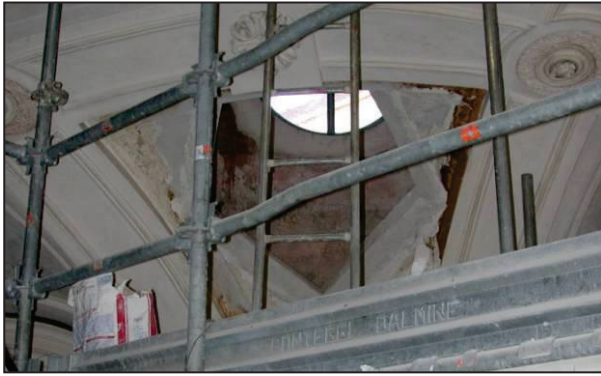
Fig. 5 - Opening of the six pentagons located in the dome above the altar after the untap the paint surface
