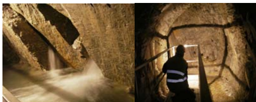
Fig. 6: On the left: Water flows from the fractured mass giving rise to the Sorgente di Tenda; on the right: Excavation face of the tapping tunnel
