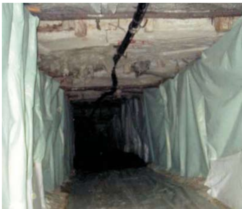
Figure 2. Scheme of the filling of a drift and photograph of a drift ready to be filled, where an impervious membrane has been installed to protect the not yet mined talc against pollution
