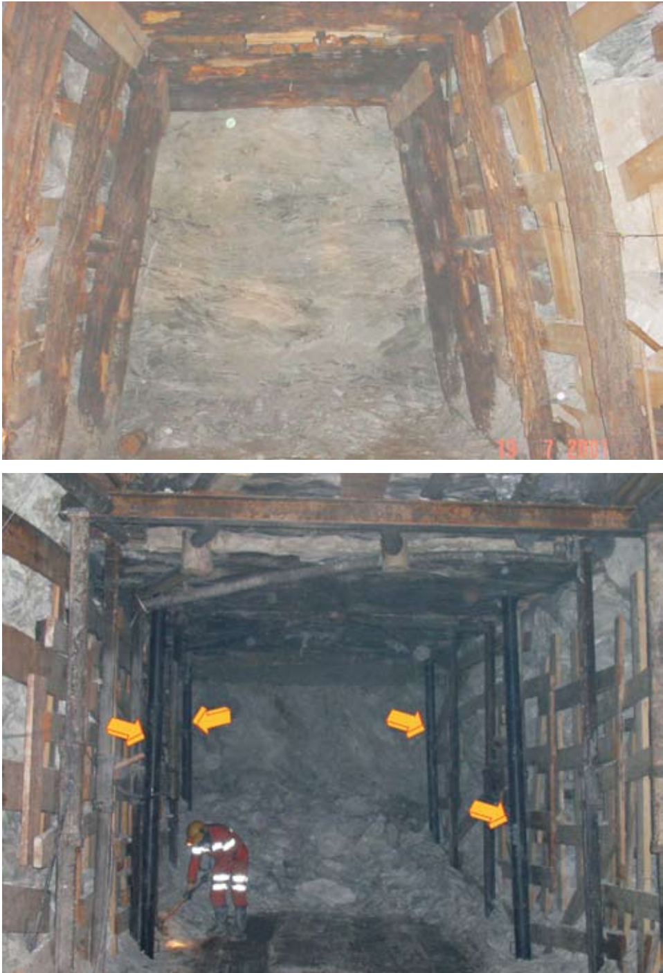
Figure 1. View of a drift supported by timber sets and hydraulic (arrows) and mechanical props
