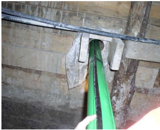
Figure 12. Detail of the installation of the assestometric casing along a transversal drift in the Rodoretto mine for a length of 26m
