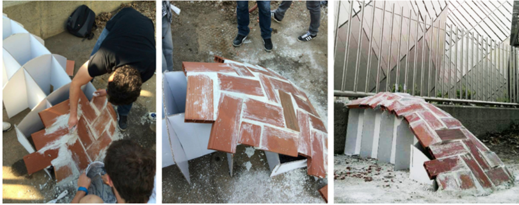
Figure 6.8: The training of brick vault construction
