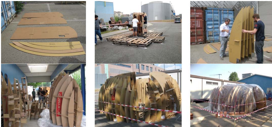
Figure 5.18: Construction of the formwork
