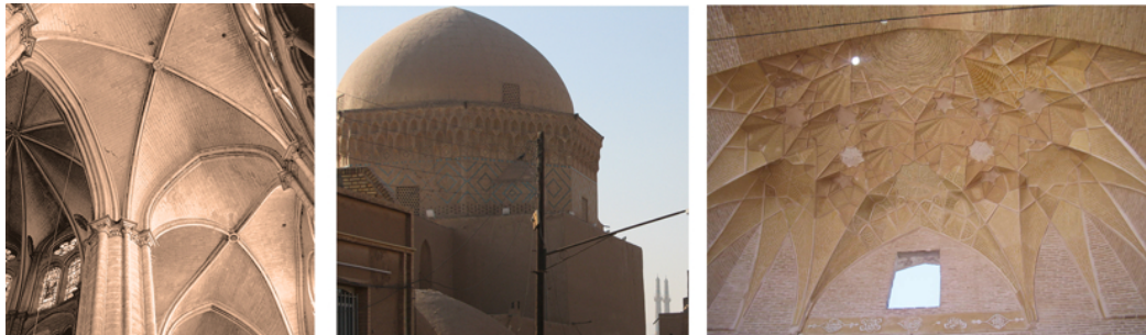
Figure 7.3: Curved surfaces constructed of bricks, a)The ambulatory roof at Bourges [40], b)The dome of Ziaiyeh School at Yazd (Autor) c)Muqarnas of Jameh Mosque and Isfahan(Autor)
