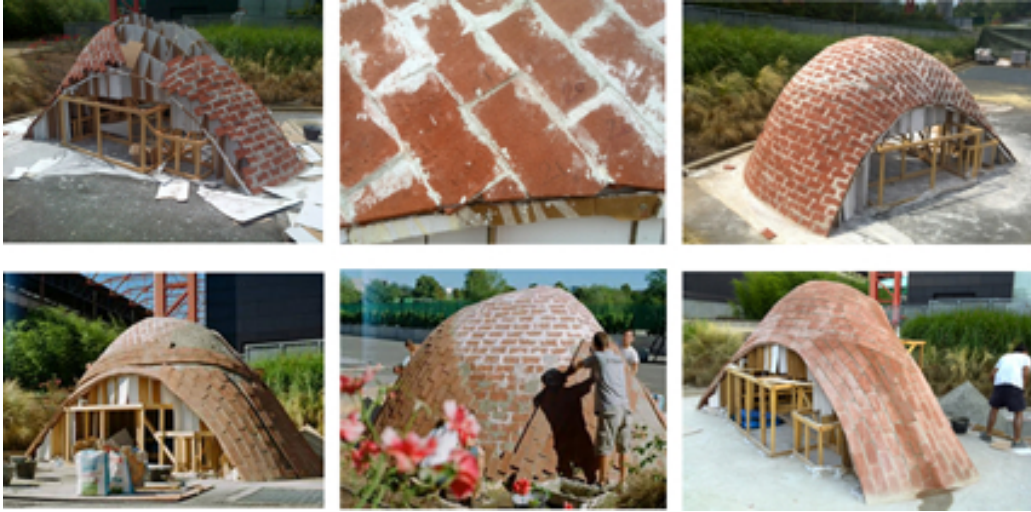
Figure 6.14: The process of constructing The Catalan Vault in workshop 2014
