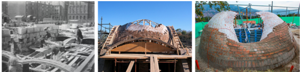
Figure 6.2: Catalan Vaults a) United States, Guastavino b)South Africa, MIT research group c) Colombia, Block research group
