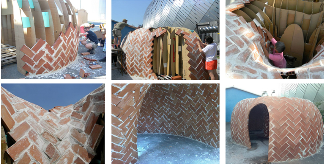
Figure 5.20: Construction Process of Brickshell
