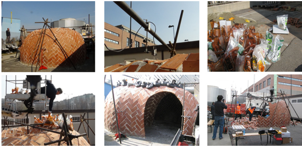
Figure 5.25: The process of Load bearing test
