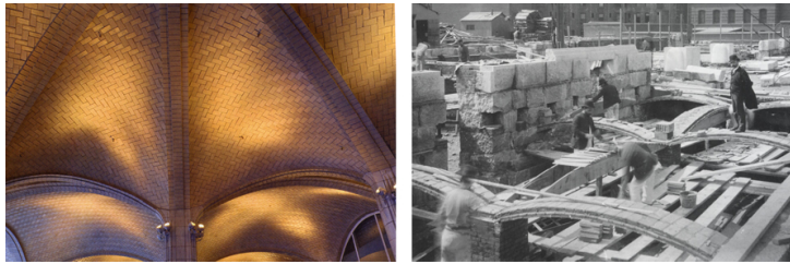
Figure 3.2: a) Tile arch supported by Ribs constructed by Guastavino b) Rafael Guastavino stranded on a newly built arch during the construction of the Boston Library, [66]
