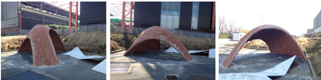
Figure 6.15: The final result of constructing The Catalan Vault in workshop 2014
