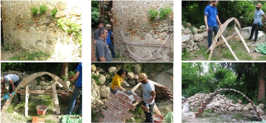
Figure 5.15: Construction of the catenary curve
