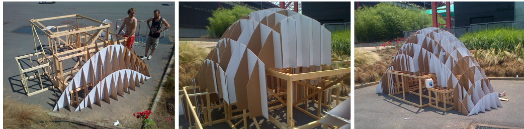
Figure 6.13: The process of the scaffolding construction
