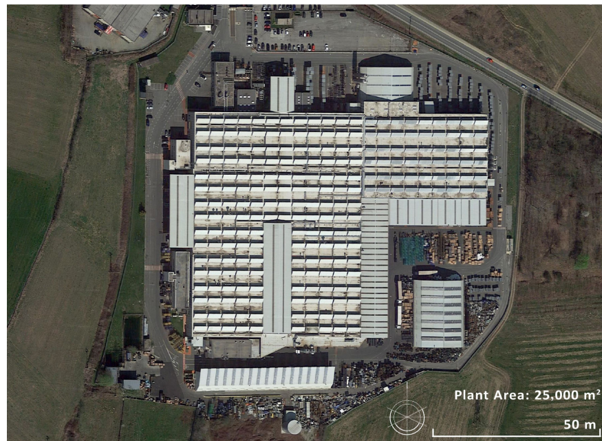
Figure 9. Case study of the industrial plant. Aerial view from Google Earth (© 2025 Google, accessed on 30 July 2025).
