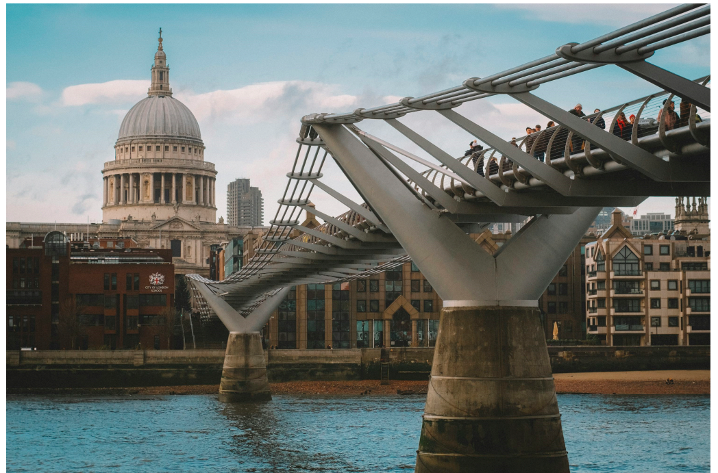
Figure 1. Millennium Bridge in London (UK) looking north.
