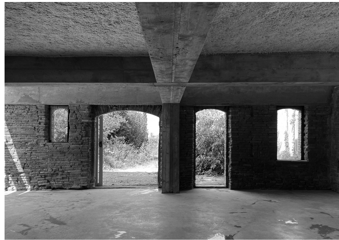
Fig. 6 - Inside, the E54 project's space is characterized by a cross-shaped reinforced concrete structure that accommodates a large community hall (Photo by BAST).
