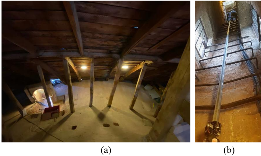
Figure 6. 12: location 5 and a detail of the steep ladder
