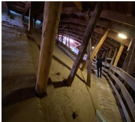
Figure 6. 13: location 6: the ramp and stairs leading to the lantern
