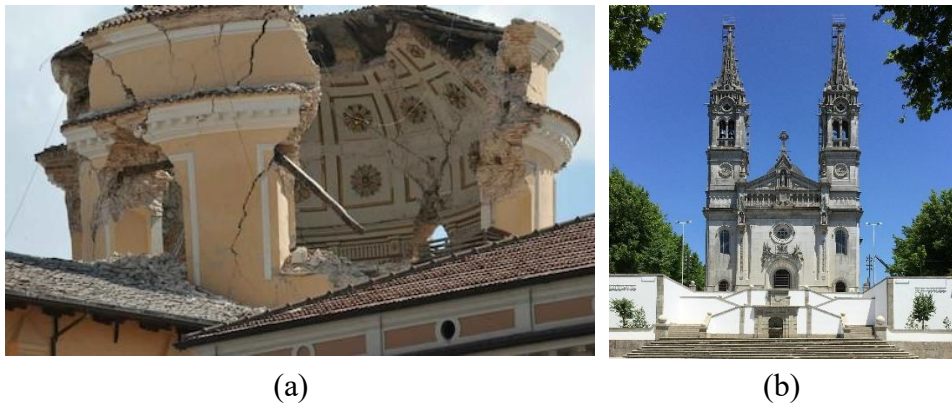
Figure 2. 7: damaged Anime Sante church and Saint Torcato church
