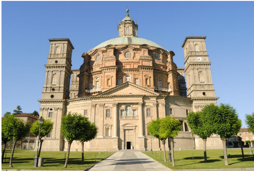
Figure 2. 10: external view of the Sanctuary of Vicoforte
