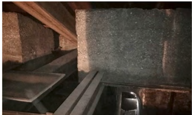
Fig. 5. Concrete blocks and coupled iron supporting beams.
