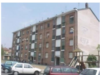
Figure 2: Photograph of the building type of the Italian apartment block (AB) built in the period 1946-60
